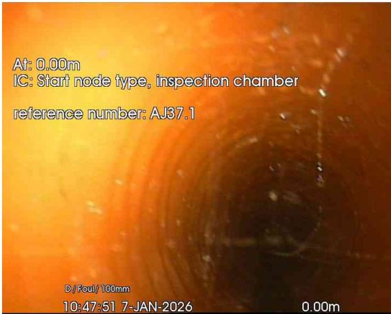
1, 00:00:01, 0.00 m Start node, inspection chamber, reference: AJ37.1
