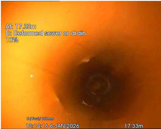
5, 00:01:10, 17.33 m Deformed sewer or drain, 10%
