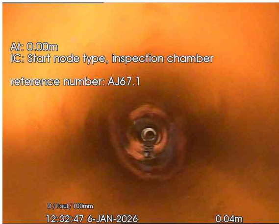
1, 00:00:01, 0.04 m Start node, inspection chamber, reference: AJ67.1
