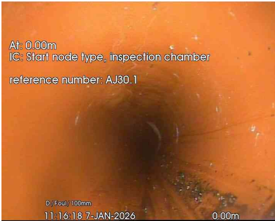
1, 00:00:01, 0.00 m Start node, inspection chamber, reference: AJ30.1
