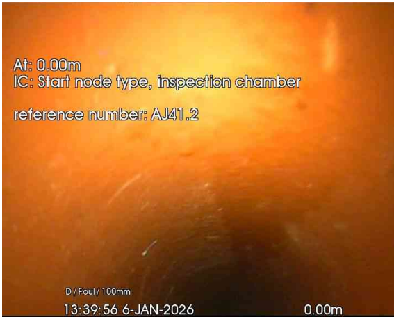
1, 00:00:01, 0.00 m Start node, inspection chamber, reference: AJ41.2
