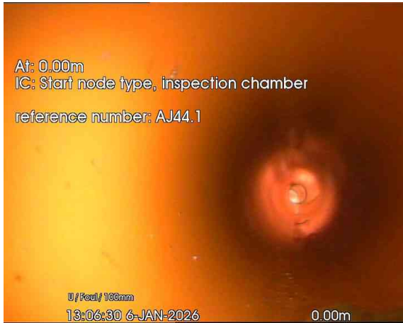
1, 00:00:01, 0.00 m Start node, inspection chamber, reference: AJ44.1
