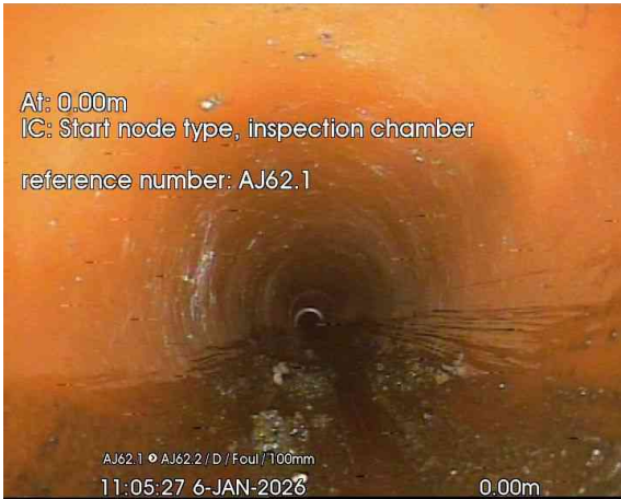
1, 00:00:00, 0.00 m Start node, inspection chamber, reference: AJ62.1
