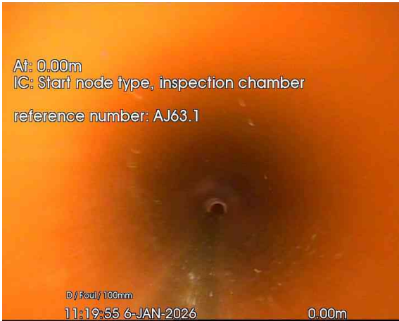
1, 00:00:01, 0.00 m Start node, inspection chamber, reference: AJ63.1
