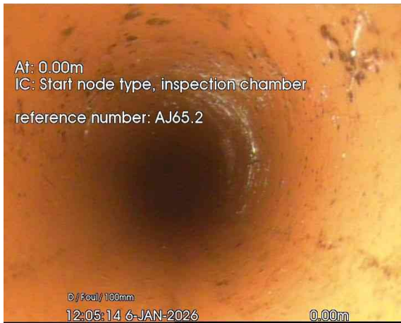
1, 00:00:01, 0.00 m Start node, inspection chamber, reference: AJ65.2
