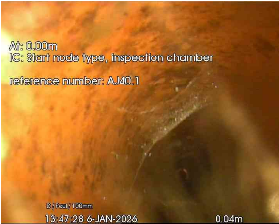
1, 00:00:02, 0.04 m Start node, inspection chamber, reference: AJ40.1
