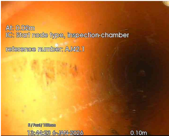
1, 00:00:01, 0.16 m Start node, inspection chamber, reference: AJ42.1
