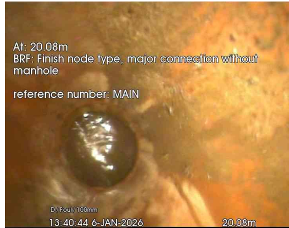
2, 00:00:44, 20.08 m Finish node, major connection without manhole, reference: MAIN
