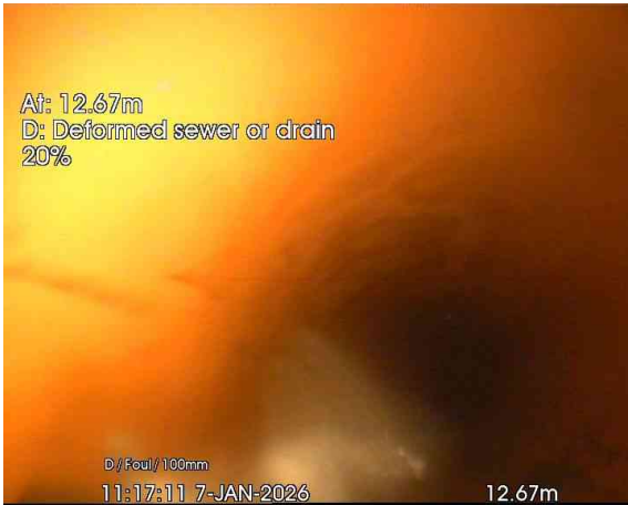
5, 00:00:35, 12.67 m Deformed sewer or drain, 20%
