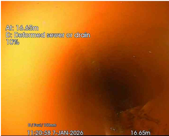
5, 00:01:16, 16.65 m Deformed sewer or drain, 10%
