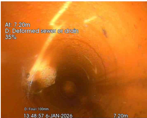
3, 00:00:18, 7.20 m Deformed sewer or drain, 35%
