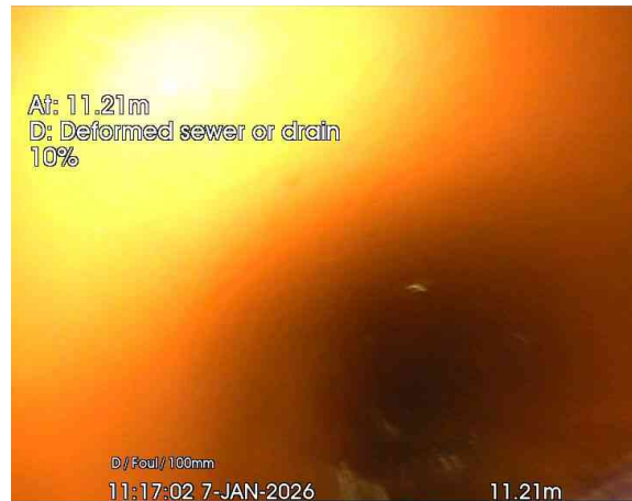
4, 00:00:30, 11.21 m Deformed sewer or drain, 10%
