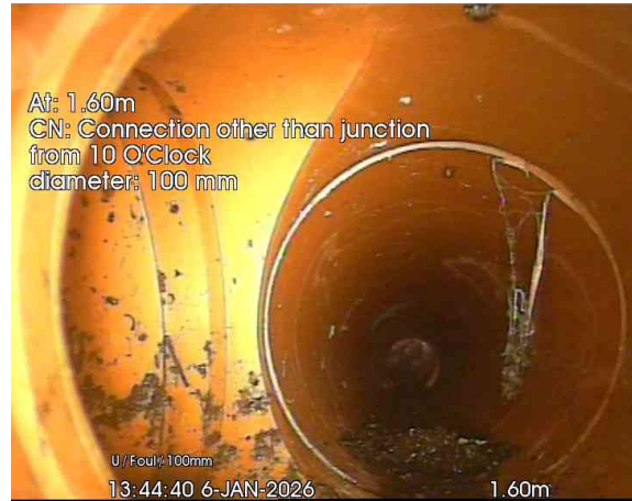
2, 00:00:08, 1.60 m Connection other than junction at 10 o'clock, 100mm dia
