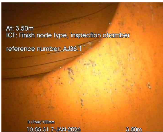
3, 00:00:15, 3.50 m Finish node, inspection chamber, reference: AJ36.1
