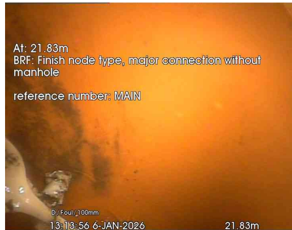
8, 00:00:55, 21.83 m Finish node, major connection without manhole, reference: MAIN
