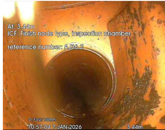
2, 00:00:10, 3.44 m Finish node, inspection chamber, reference: AJ36.2
