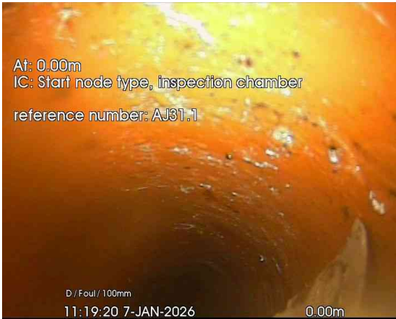
1, 00:00:01, 0.00 m Start node, inspection chamber, reference: AJ31.1
