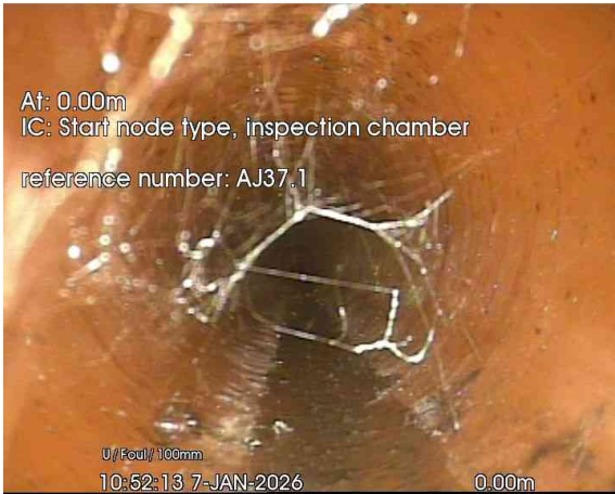
1, 00:00:01, 0.00 m Start node, inspection chamber, reference: AJ37.1
