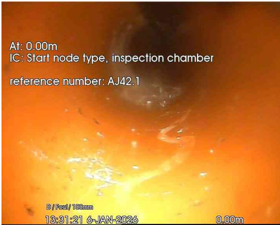
1, 00:00:01, 0.00 m Start node, inspection chamber, reference: AJ42.1
