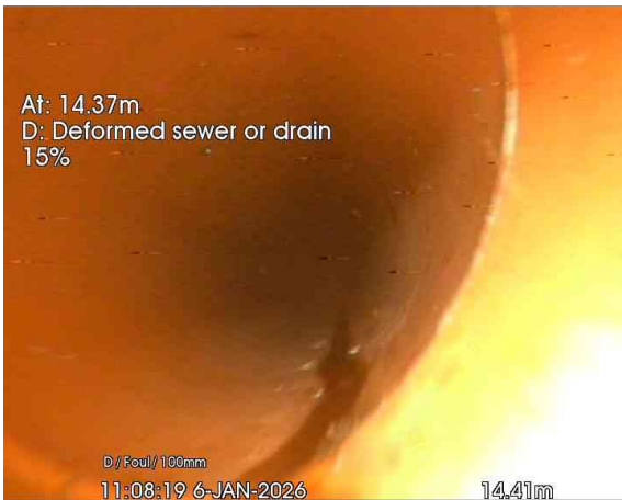
3, 00:00:28, 14.41 m Deformed sewer or drain, 15%
