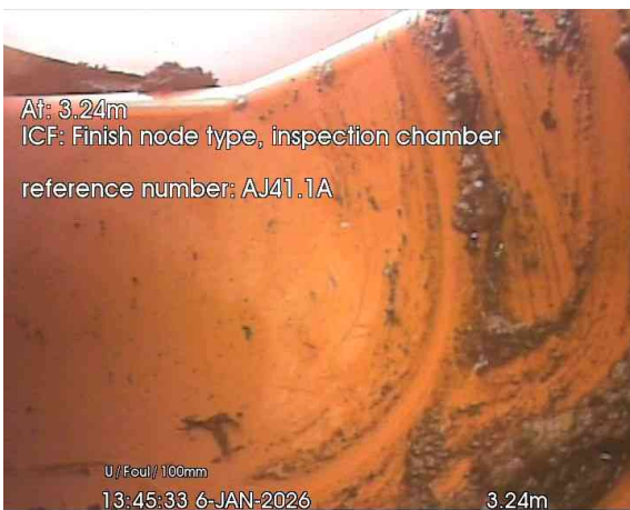
3, 00:00:26, 3.24 m Finish node, inspection chamber, reference: AJ41.1A
