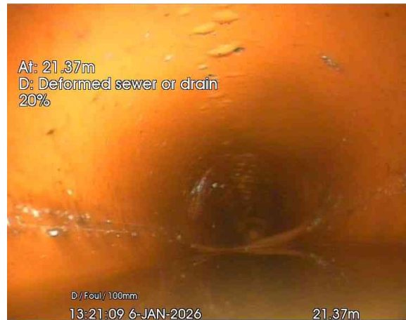
4, 00:01:01, 21.37 m Deformed sewer or drain, 20%
