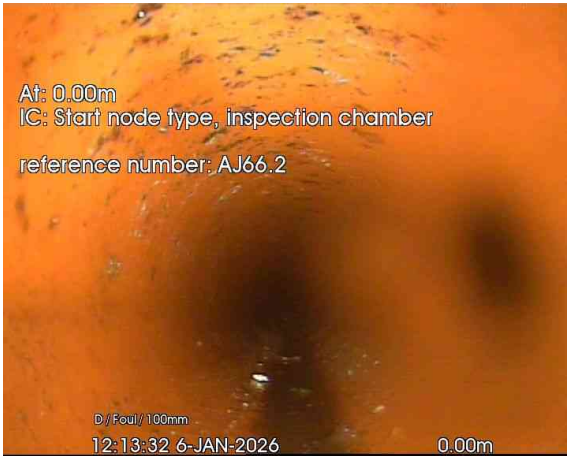
1, 00:00:01, 0.00 m Start node, inspection chamber, reference: AJ66.2
