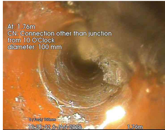
2, 00:00:12, 1.76 m Connection other than junction at 10 o'clock, 100mm dia
