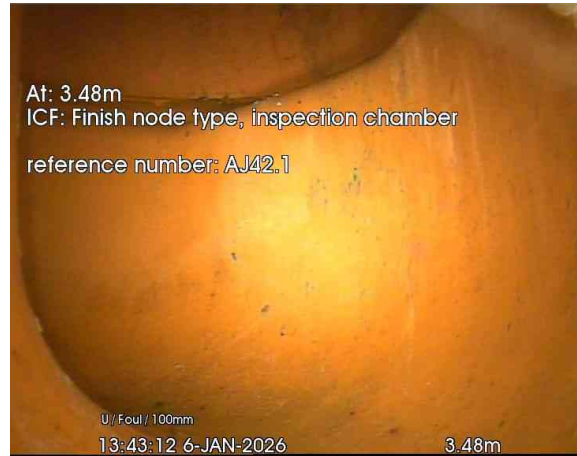
2, 00:00:12, 3.48 m Finish node, inspection chamber, reference: AJ42.1
