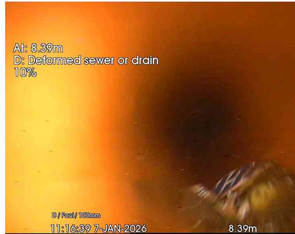
2, 00:00:17, 8.39 m Deformed sewer or drain, 10%
