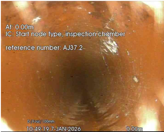
1, 00:00:00, 0.00 m Start node, inspection chamber, reference: AJ37.2
