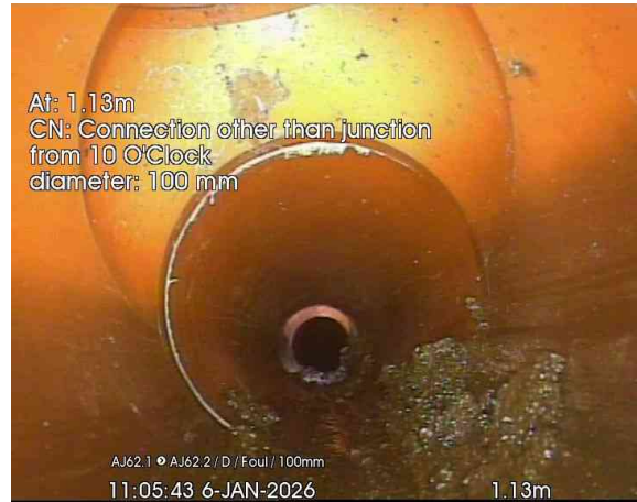
2, 00:00:07, 1.13 m Connection other than junction at 10 o'clock, 100mm dia
