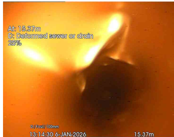
4, 00:01:18, 15.37 m Deformed sewer or drain, 25%
