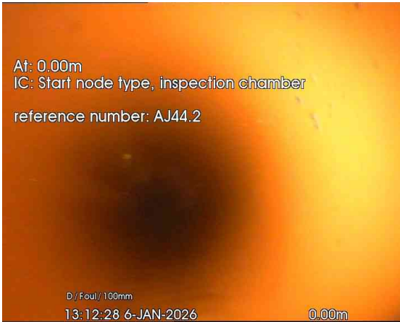
1, 00:00:01, 0.00 m Start node, inspection chamber, reference: AJ44.2
