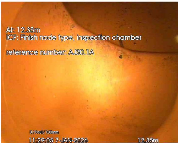
3, 00:00:25, 12.35 m Finish node, inspection chamber, reference: AJ30.1A
