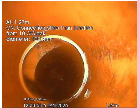
2, 00:00:08, 1.27 m Connection other than junction at 10 o'clock, 100mm dia
