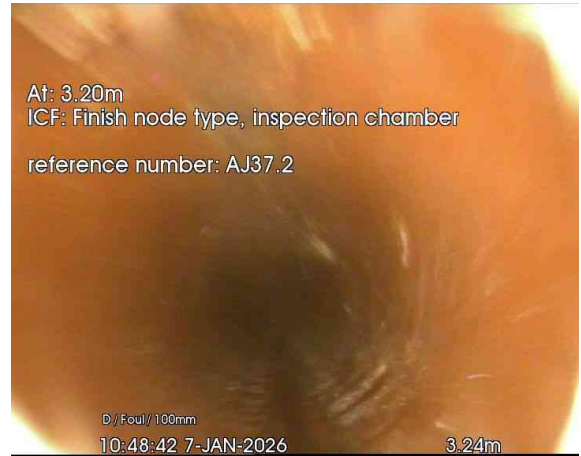
2, 00:00:17, 3.27 m Finish node, inspection chamber, reference: AJ37.2
