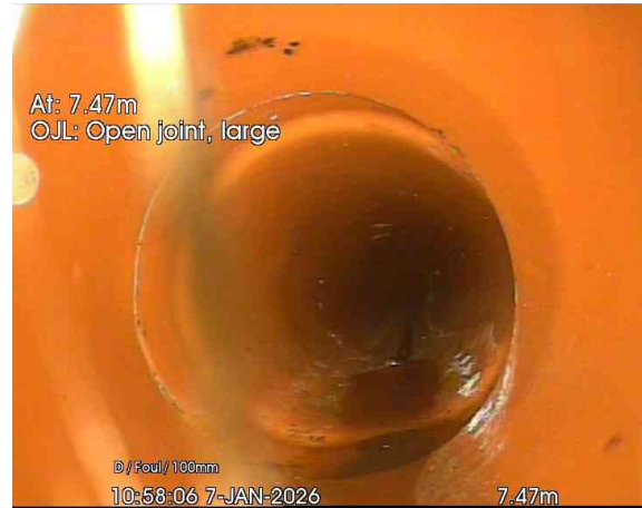
2, 00:00:17, 7.47 m Open joint, large
