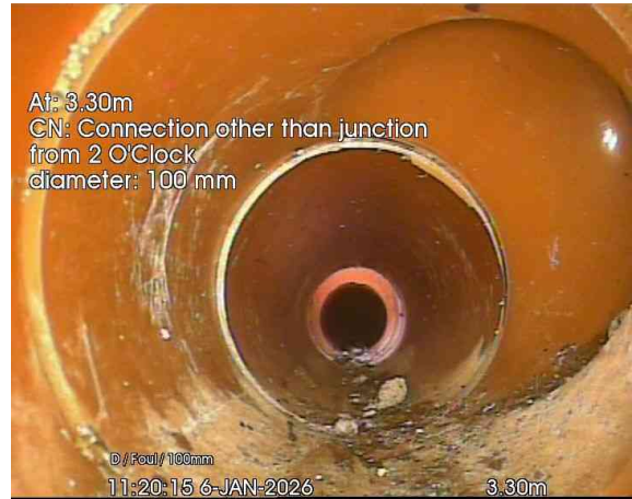
2, 00:00:12, 3.30 m Connection other than junction at 2 o'clock, 100mm dia
