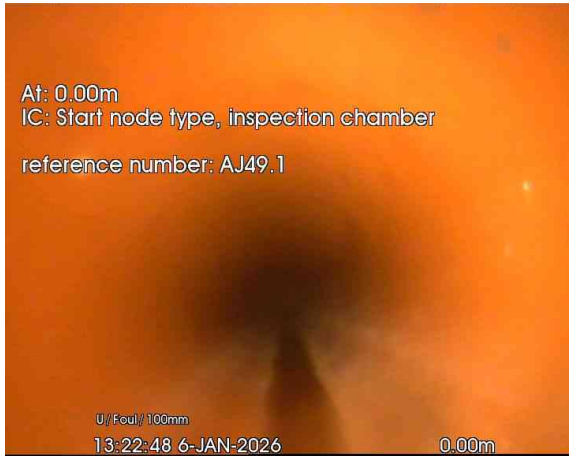
1, 00:00:01, 0.00 m Start node, inspection chamber, reference: AJ49.1
