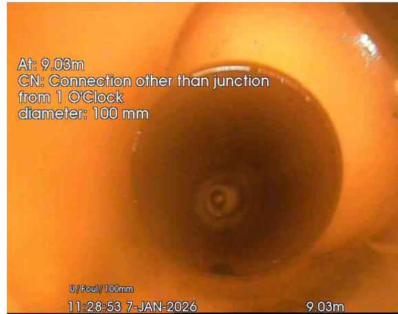
2, 00:00:19, 9.03 m Connection other than junction at 1 o'clock, 100mm dia
