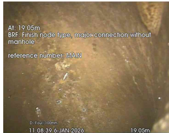
4, 00:00:41, 19.05 m Finish node, major connection without manhole, reference: MAIN
