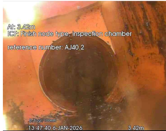
2, 00:00:09, 3.42 m Finish node, inspection chamber, reference: AJ40.2
