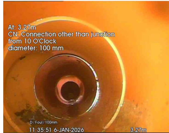
2, 00:00:14, 3.27 m Connection other than junction at 10 o'clock, 100mm dia
