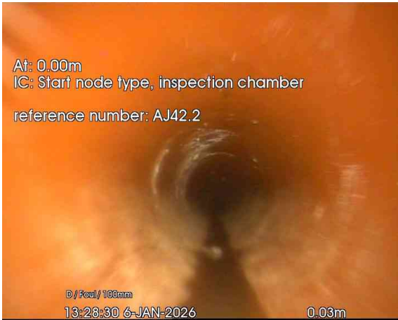
1, 00:00:01, 0.03 m Start node, inspection chamber, reference: AJ42.2
