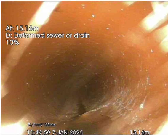
3, 00:00:31, 15.16 m Deformed sewer or drain, 10%
