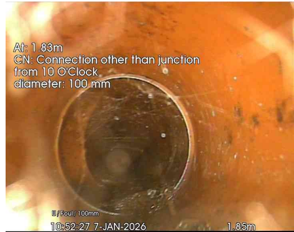
2, 00:00:07, 1.85 m Connection other than junction at 10 o'clock, 100mm dia
