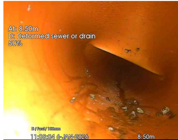
2, 00:00:18, 8.50 m Deformed sewer or drain, 50%
