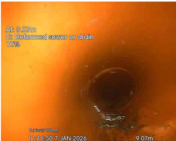
3, 00:00:23, 9.07 m Deformed sewer or drain, 10%
