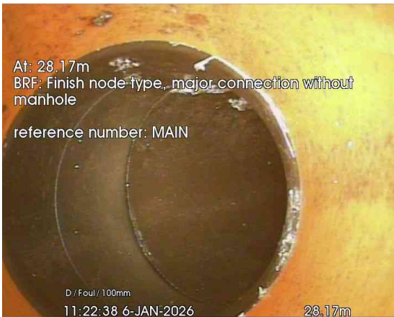
3, 00:01:06, 28.17 m Finish node, major connection without manhole, reference: MAIN
