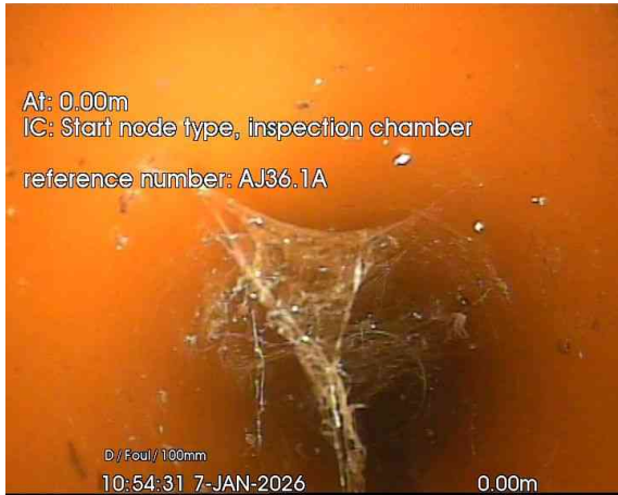
1, 00:00:01, 0.00 m Start node, inspection chamber, reference: AJ36.1A
