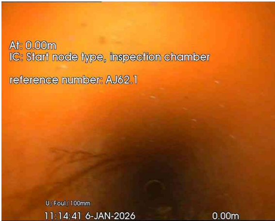
1, 00:00:01, 0.00 m Start node, inspection chamber, reference: AJ62.1
