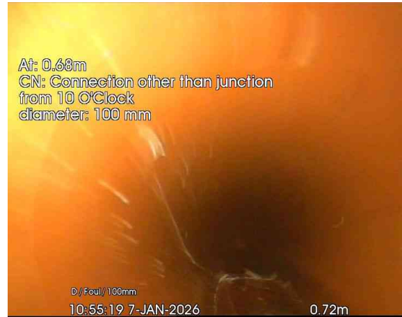
2, 00:00:10, 0.72 m Connection other than junction at 10 o'clock, 100mm dia
