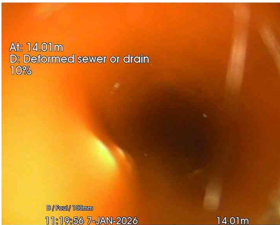
3, 00:00:28, 14.01 m Deformed sewer or drain, 10%
