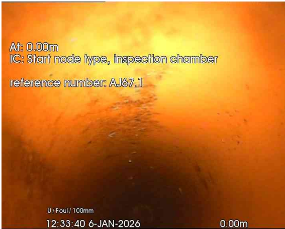
1, 00:00:01, 0.00 m Start node, inspection chamber, reference: AJ67.1
