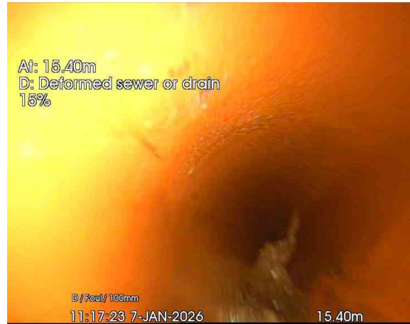
6, 00:00:43, 15.40 m Deformed sewer or drain, 15%
