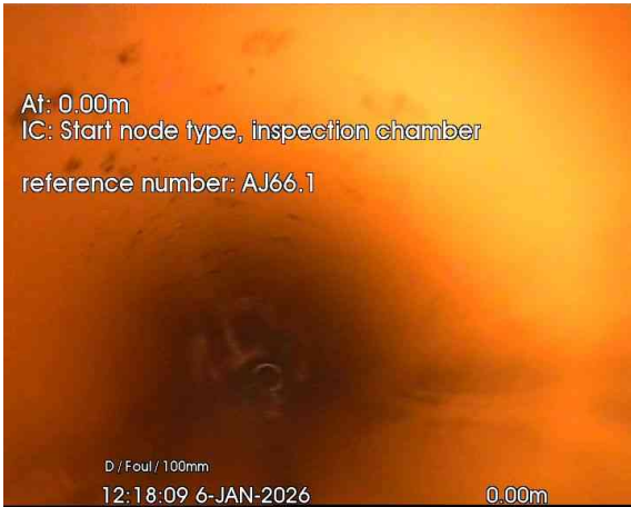
1, 00:00:01, 0.00 m Start node, inspection chamber, reference: AJ66.1
