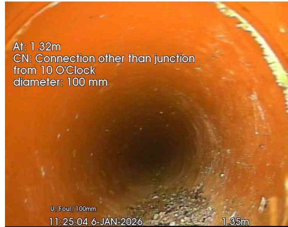
2, 00:00:04, 1.35 m Connection other than junction at 10 o'clock, 100mm dia
