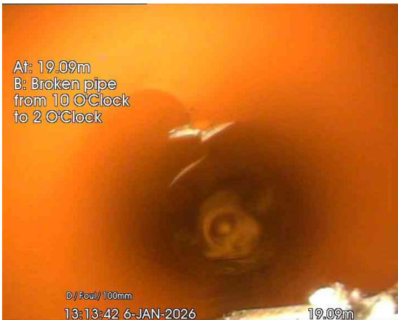
7, 00:00:46, 19.09 m Broken pipe from 10 o'clock to 2 o'clock
