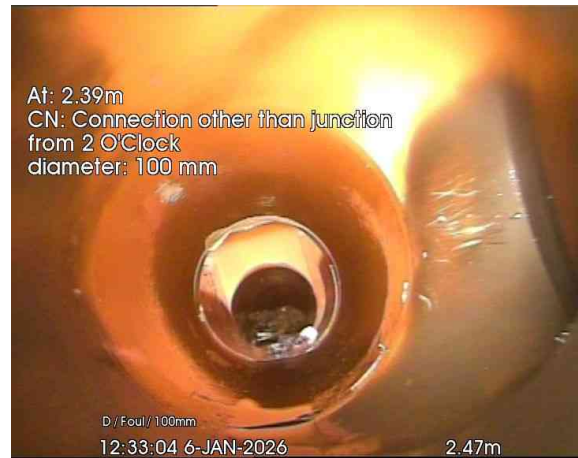
2, 00:00:09, 2.56 m Connection other than junction at 2 o'clock, 100mm dia
