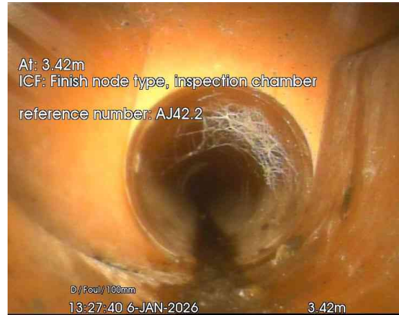
2, 00:00:13, 3.42 m Finish node, inspection chamber, reference: AJ42.2
