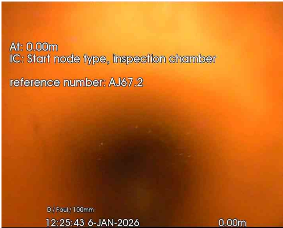
1, 00:00:01, 0.00 m Start node, inspection chamber, reference: AJ67.2
