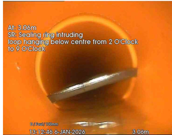
2, 00:00:08, 3.06 m Sealing ring intruding, loop hanging below centre from 2 o'clock to 9 o'clock
