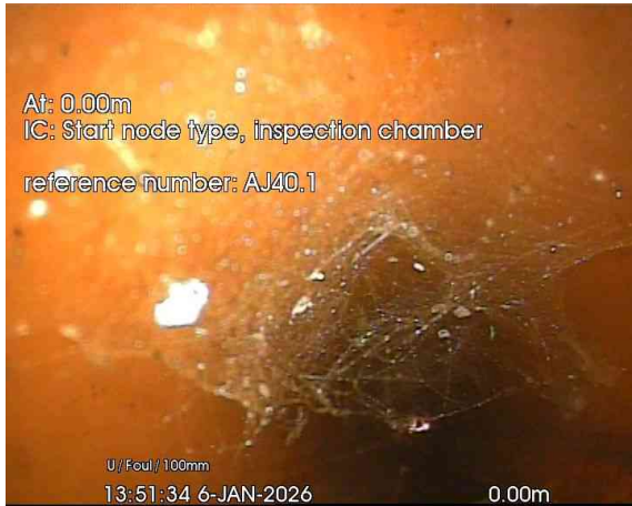
1, 00:00:03, 0.00 m Start node, inspection chamber, reference: AJ40.1
