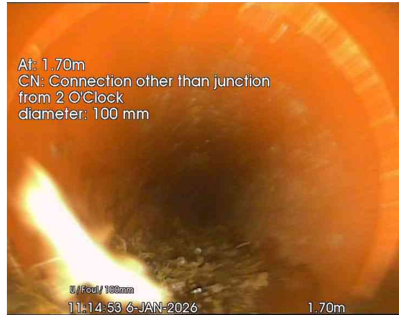
2, 00:00:06, 1.70 m Connection other than junction at 2 o'clock, 100mm dia
